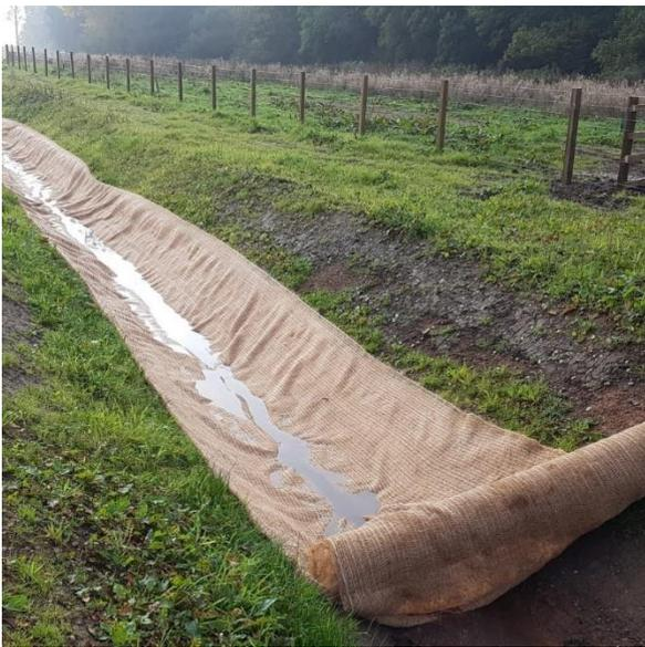
It is important that silt fencing and other pollution protection measures are regularly inspected, sediment removed and systems maintained to ensure ongoing efficiency. This infrastructure should therefore be inspected by the ECoW on a daily basis and any flaws / failures reported to the main contractor. Works should not proceed unless all measures are in place to the satisfaction of the ECoW.
