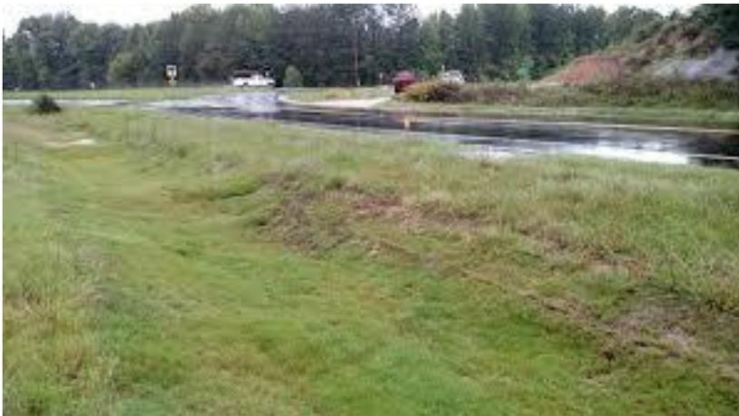
A swale is an elongate vegetated drainage channel designed to capture runoff drainage from upgradient areas of the construction site. The swale is designed to encourage / maximise infiltration of runoff waters through the permeable base / sides as it is transferred to the end point of the swale. The swale is vegetated to provide attenuation of sediment and other pollutants which may be present and therefore also comprises a source-control treatment step.
